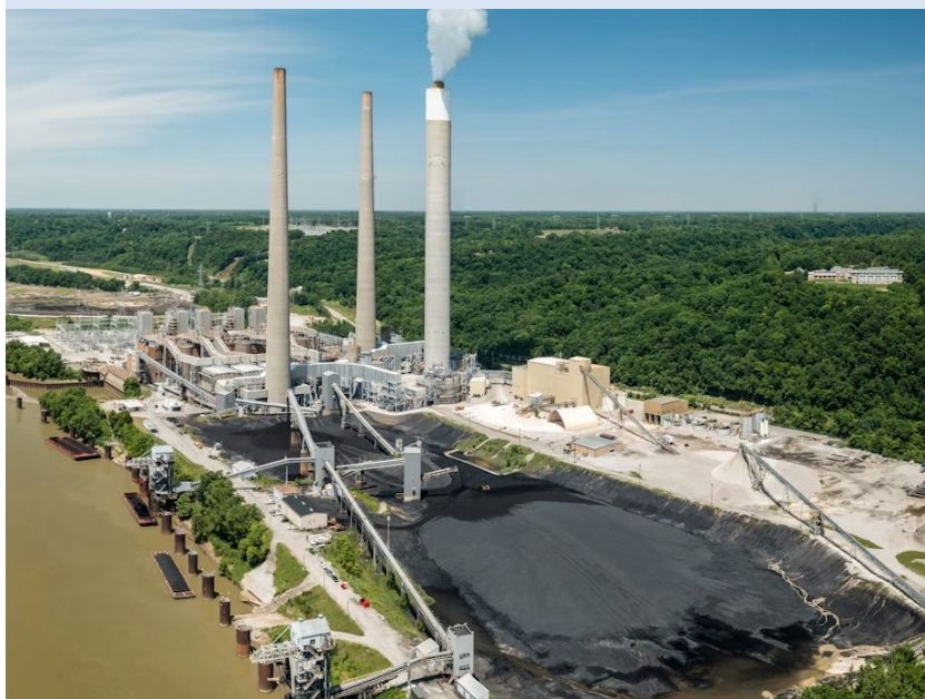
Aerial view of a coal-fired power plant near Ohio. Photo: Shutterstock.
