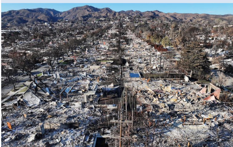
An aerial view of homes destroyed in the Palisades Fire, in Pacific Palisades, California. Photo: Mario Tama/Getty Images.
