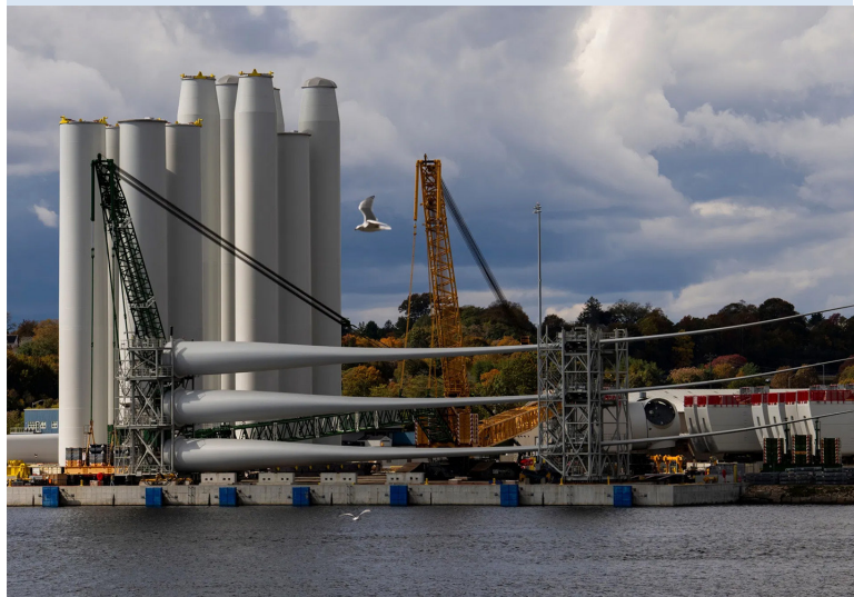
Wind turbine tower sections and blades at the Revolution Wind project assembly site in New London, Connecticut. Photo credit: Joe Buglewicz/Bloomberg.
