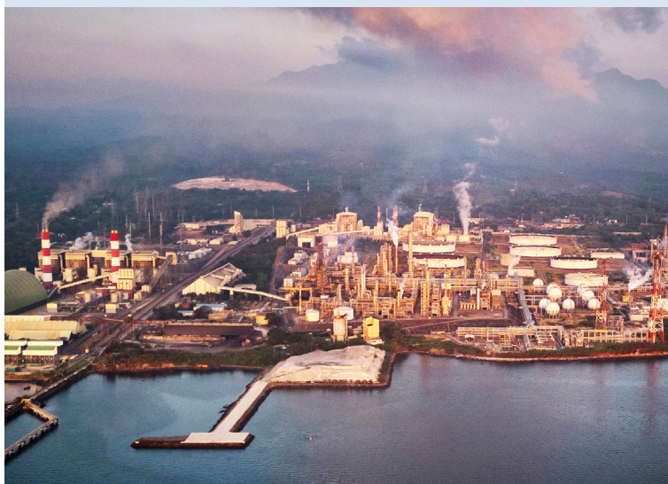
The Petron oil refinery in the Philippines, which received crude oil from Russia as countries scramble for alternatives to disrupted Middle Eastern supplies. Photo: Ezra Acayan/Getty Images.
